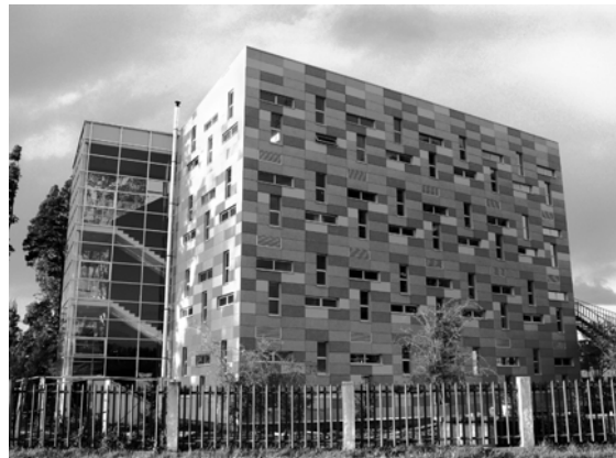
Figure 1: View of the Multi-Media Building from the South
