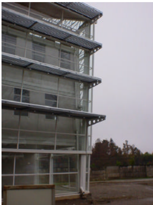
Figure 7: Overhang on the north facade
