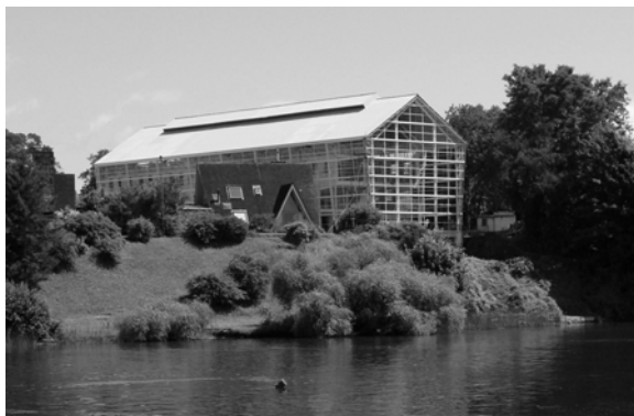
Figure 1 : View of southern and eastern facade from across the river
